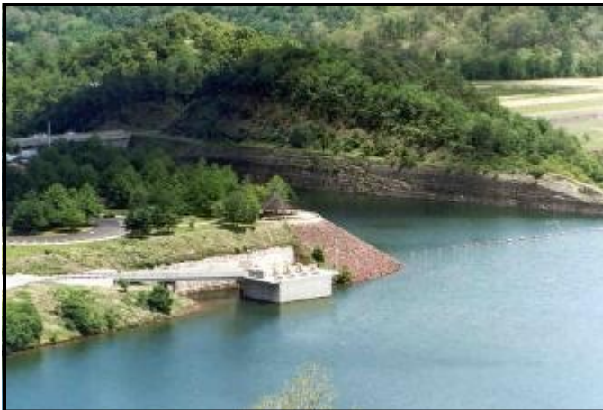
Our main source of renewable electricity: the certified, low-impact facility of the Raystown Hydroelectric Project, Juniata River, Huntingdon County, PA (photo courtesy of www.lowimpacthydro.org )
